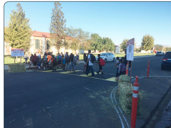
Hay bales, spray paint, and traffic cones are used to create curb extensions to narrow the street in order to slow traffic and shorten the crossing distance for people walking. The temporary crosswalk makes it clear that children will be crossing the street here to reach their school. Photo: Alta Planning + Design
