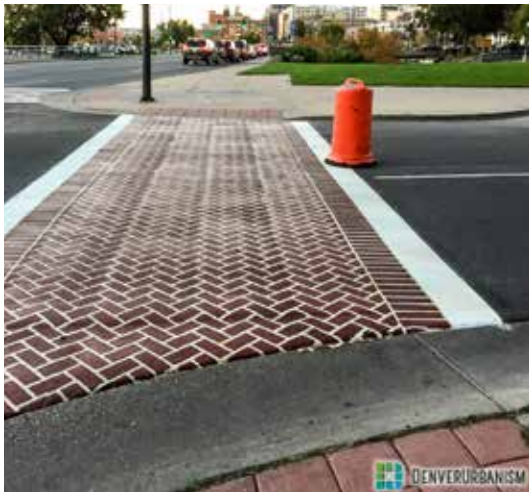
Thermoplastic faux-brick pavers are eye catching. The durable material does not typically fade over time and is longer-lasting than paint (Image: Denver Urbanism).
