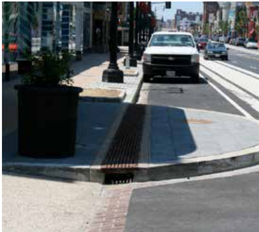
Curb extension with drainage inlet, artistic stamped concrete, brick paving, and planter (Image: Eric Fidler, https://www.flickr.com/photos/greatphotographic/5996098479 ).
