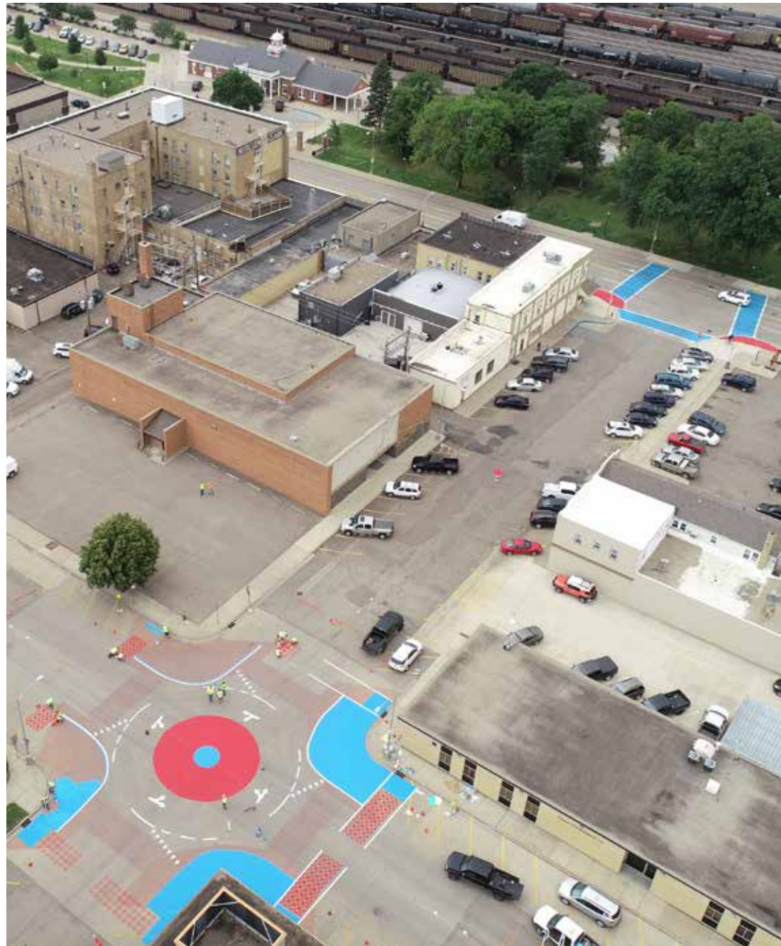
Drone footage of the project installation (Image: Houston Engineering / City of Mandan).
