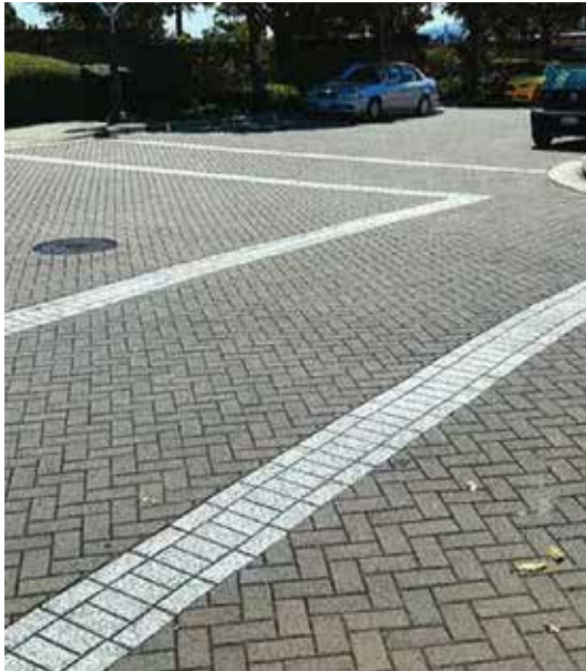
Interlocking pavers form an attractive streetscaping element. Note that reflective, 12" wide crosswalk striping is recommended in thermoplastic instead of brick (image: interlockdesign.org)
