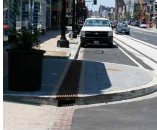
Curb extension with drainage inlet, artistic stamped concrete, brick paving, and planter (Image: Eric Fidler, https://www.flickr.com/photos/greatphotographicon/5996098479 ).
