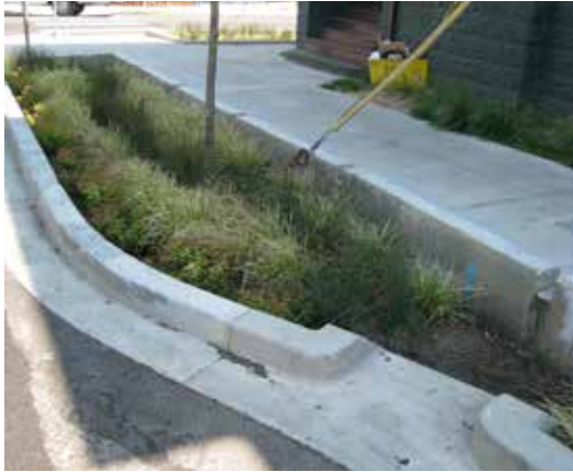
This curb extension doubles as a bioswale to filter stormwater (Image: Alta Planning + Design).
