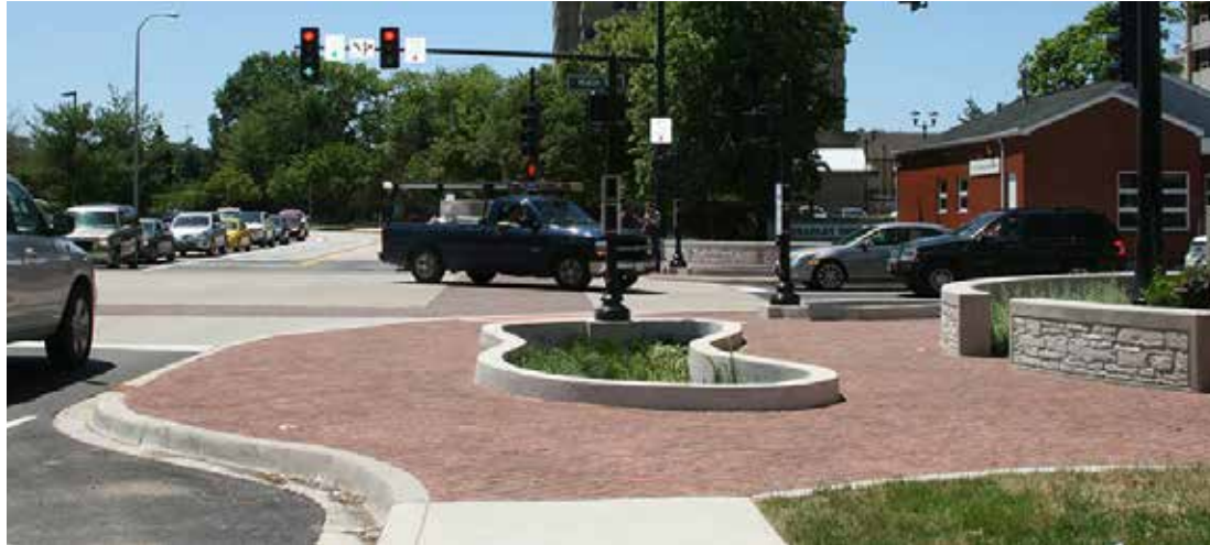
Curb extensions with decorative brick, stormwater features, and a low ledge that doubles as seating (image: Induced.info).
