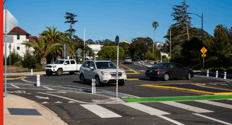
Mini roundabout in California reduces speeds.
